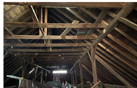
Interior of the barn's loft and rafters, courtesy of Ryan Cutting
