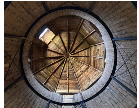
Interior of Cleveland Barn silo. Photo courtesy of Ryan Cutter.
