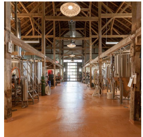
Timber framing inside the barn. Photo courtesy of Throwback Brewery
