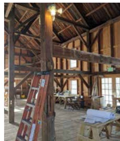
Recent interior renovation work underway.
