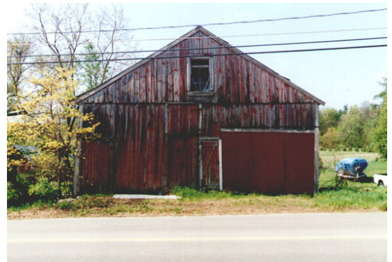
Lawrence Barn gable end prior to renovation courtesy of the town of Hollis
