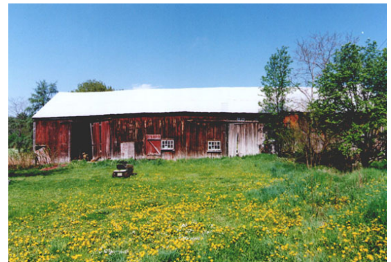
Lawrence Barn prior to renovation courtesy of the town of Hollis
